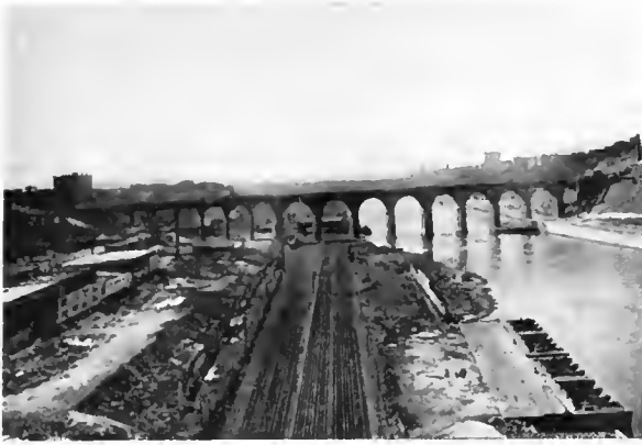
ANOTHER VIEW OF HIGH BRIDGE SHOWING RAILROAD TRACKAGE PARALLELING WATERWAY.
